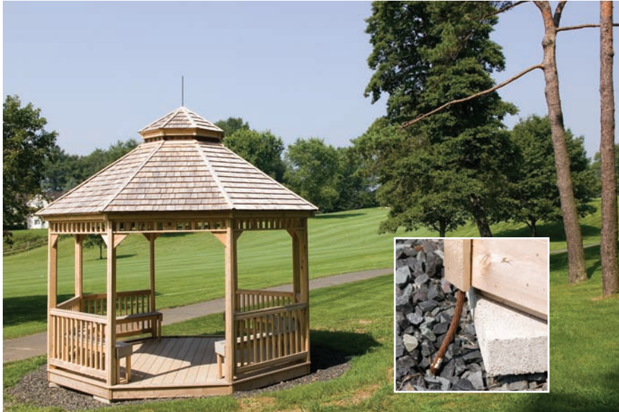
Bollinger encourages courses to install defibrillators around the course, in the clubhouse and maintenance shop. Additional recommended safety installations include UL approved lightning shelters, which incorporate multiple grounding straps (shown in inset photo).
